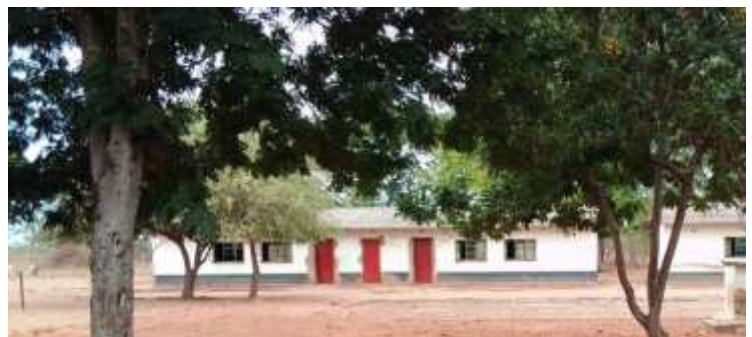
Hwata Secondary – July 2022, after repairs
